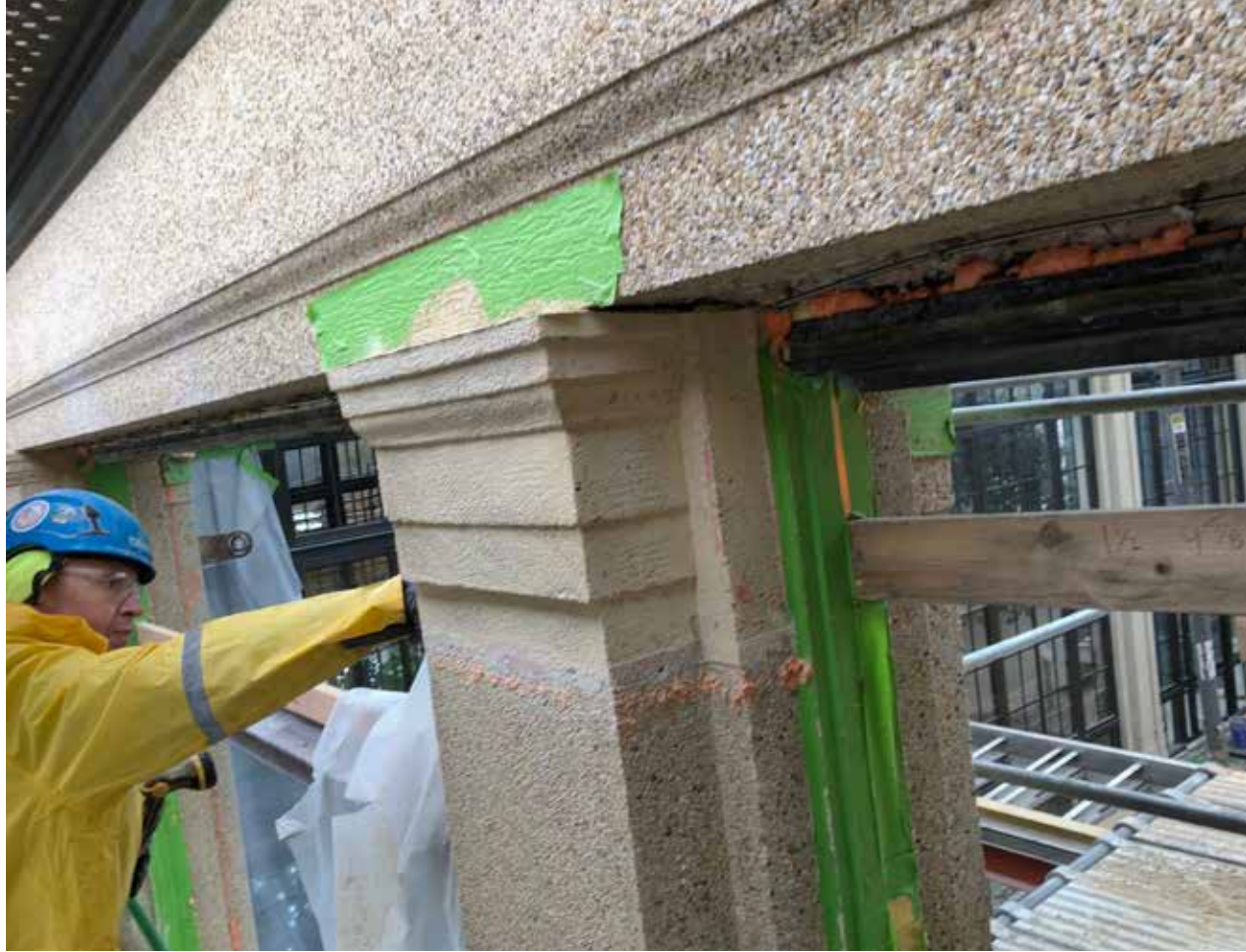
Left: Reproducing mosaic concrete required evaluating materials, molds, placement, and finishes. These precast mosaic concrete samples were evaluated onsite to assure consistency of appearance. Photo by Hank Davis.
