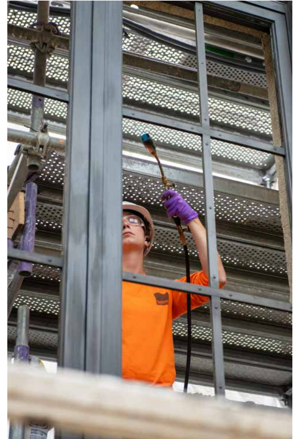
Left: Prone to discoloration and corrosion, bronze features of the Orchid House were repaired and restored. Bronze features on the north side of the building were replaced to accommodate architectural changes. Photo courtesy of John Milner Architects, Inc.
