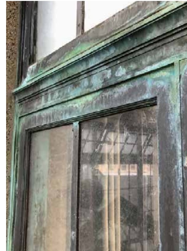
Left: Prone to discoloration and corrosion, bronze features of the Orchid House were repaired and restored. Bronze features on the north side of the building were replaced to accommodate architectural changes. Photo courtesy of John Milner Architects, Inc.
